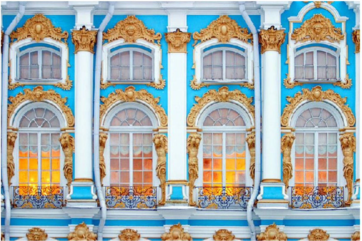
Facade decoration of Catherine Palace in Tsarskoye Selo
